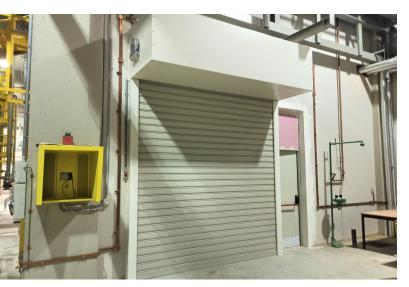
Fire rolling shutters SAFEROLL EI60 offer an excellent solution for separating fire compartments in areas with a flammable environment and are ideal for use on protected escape routes.
